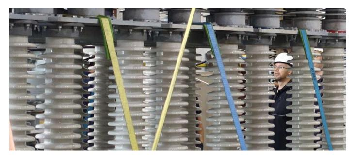
In HVDC substations, a considerable number of switching components are installed. In the 2017 CIGRE Technical Brochure "Technical Requirements and Specifications of State-of-the-Art HVDC Switching Equipment", no less than 24 types of HVDC switchgear are identified, each with a different functionality.
